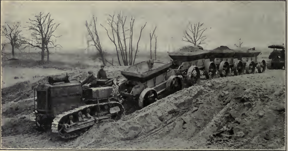
HOLT CATERPILLAR TRACTOR HAULING TROY TRAILERS IN THE CONSTRUCTION OF THE VICTORY MEMORIAL DRIVE BY THE BOARD OF PARK COMMISSIONERS OF MINNEAPOLIS, MINNESOTA
